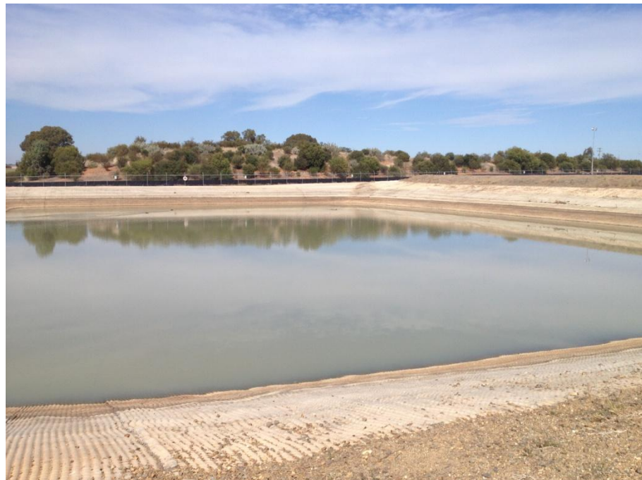
UPS Stormwater Collection Pond
