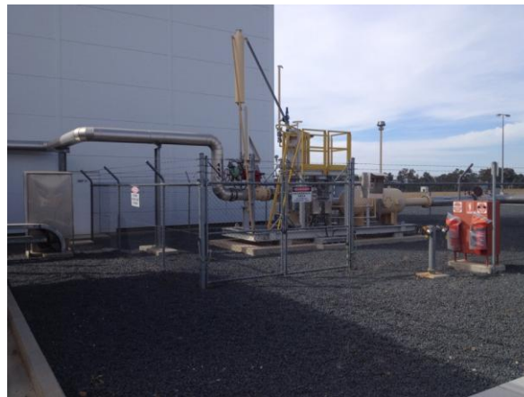
UPS Final Gas Filters
