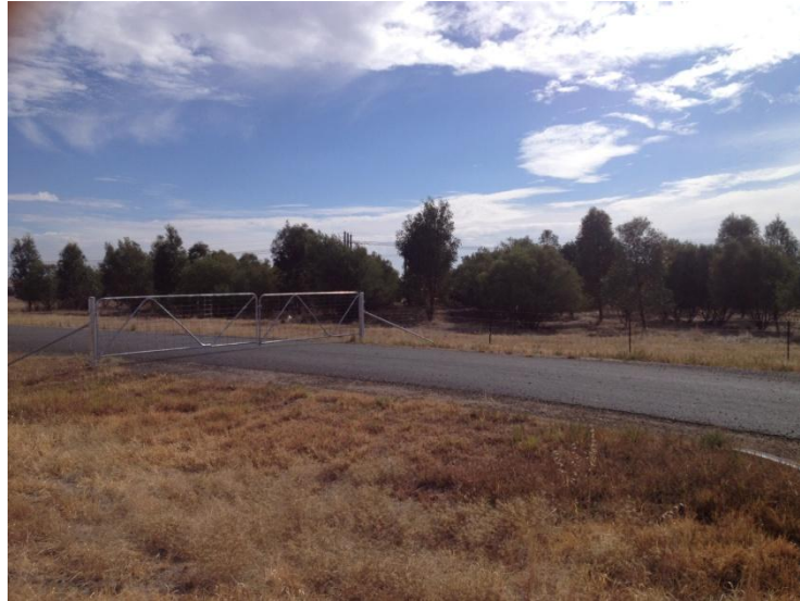
UPS Landscaping near Switchyard
