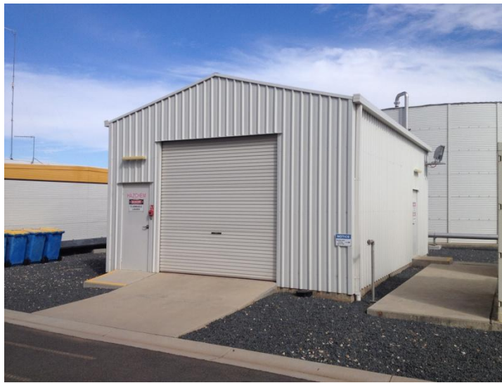
UPS Hazardous Chemical Building
