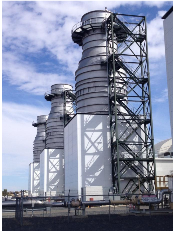
UPS Emission Stacks
