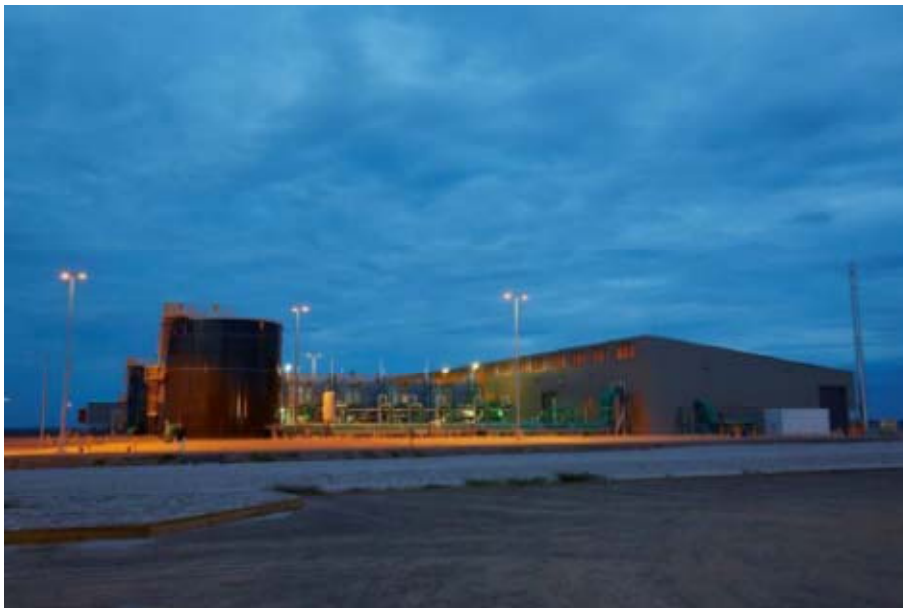
Reedy Creek Water Treatment Facility
