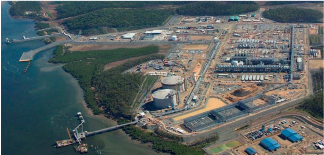
Curtis Island overview
