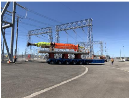
Old rotor being removed at Mortlake
