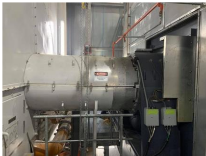
Final stages of commissioning
