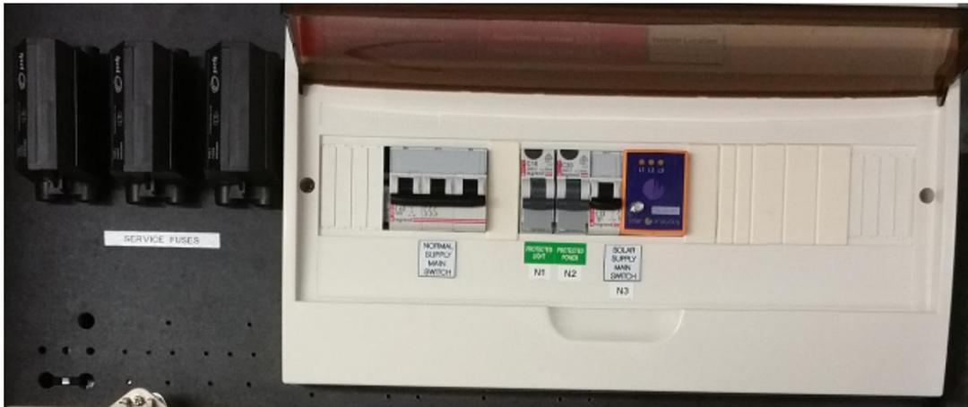
*Figure 3 Solar Smart Monitor in Main Load Centre on DB*
