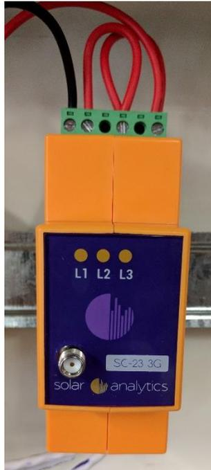
*Figure 5 SC-23 with 1-phase tail in DIN rail*
