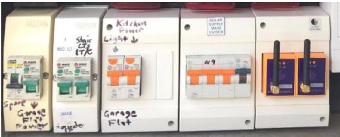
Figure 2 Solar Smart Monitor in separate DIN Enclosure
