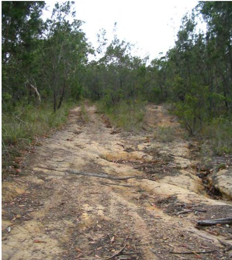
Plate 7-7: Similar to Plate 7-4, this photograph shows a heavily eroding road in Transect 5, looking northeast. Note the exposed bedrock in the right foreground, indicating the soil profile in this area is very thin.
