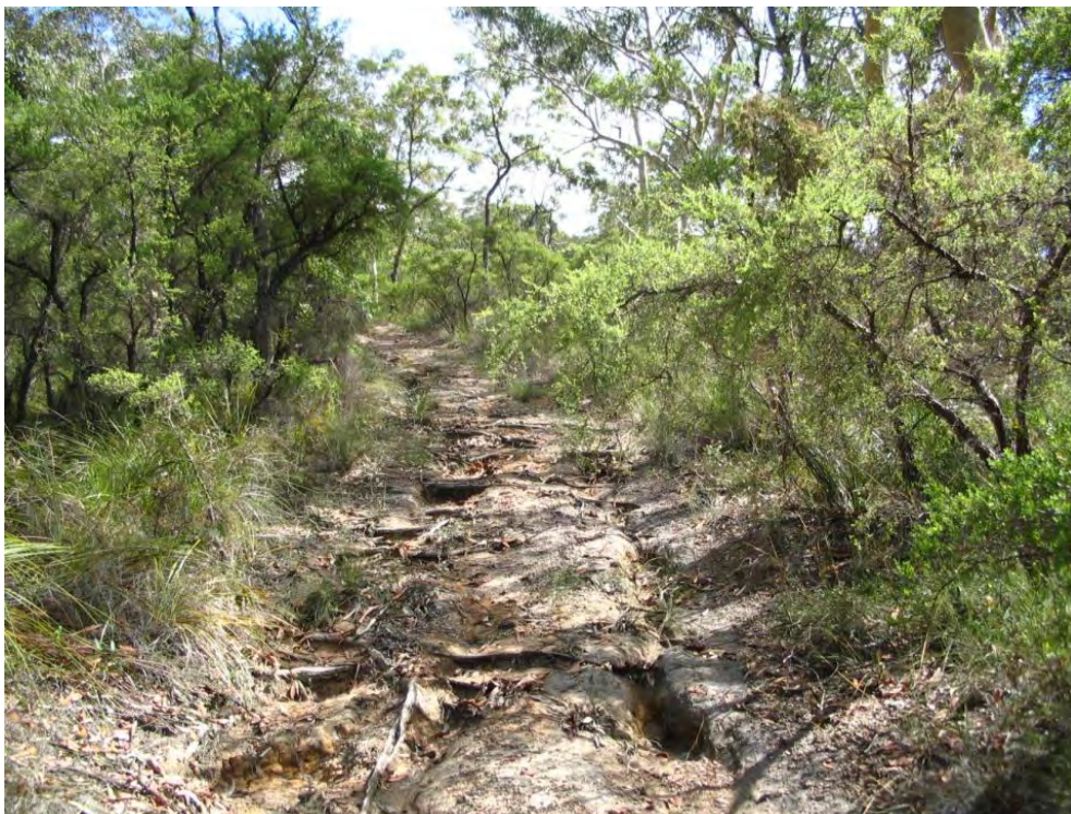
Plate 7-5: Transect 1 looking north. This road reveals the extent of erosion occurring without vegetation cover. Note the rilling down the road. It should be noted that numerous forest fires have occurred in this area, and it is likely that much of the study area would have been cleared and looked similar to this road.
