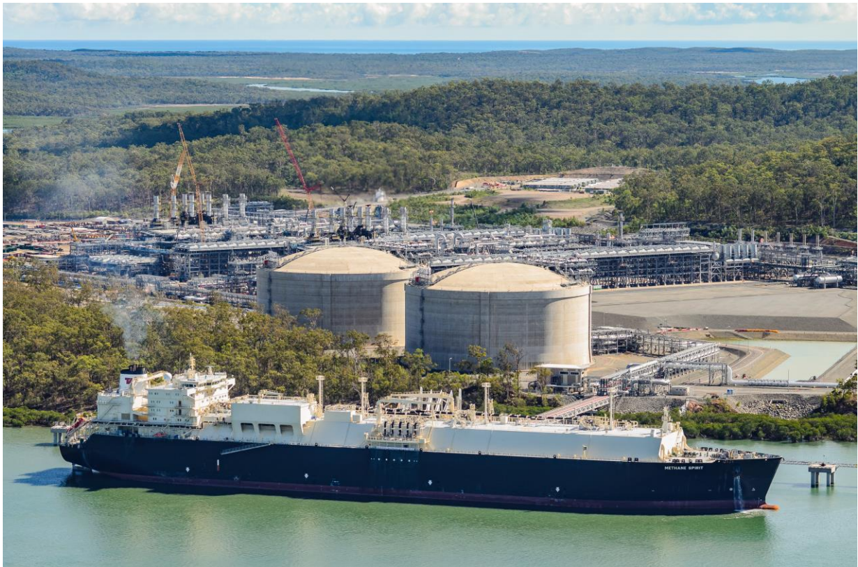
Australia Pacific LNG facility on Curtis Island
