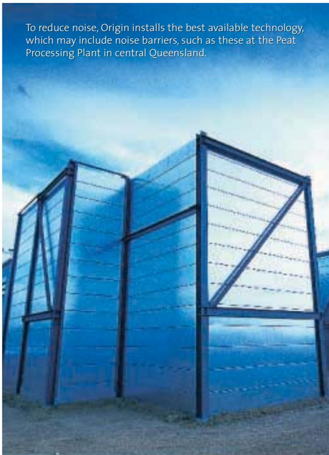
To reduce noise, Origin installs the best available technology, which may include noise barriers, such as these at the Peat Processing Plant in central Queensland.
