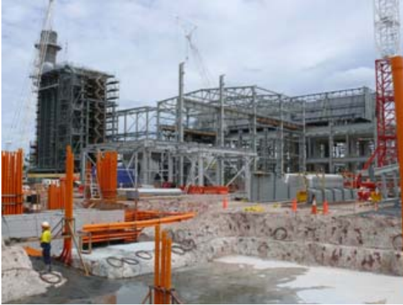
Darling Downs PS Turbine Building steel erection
