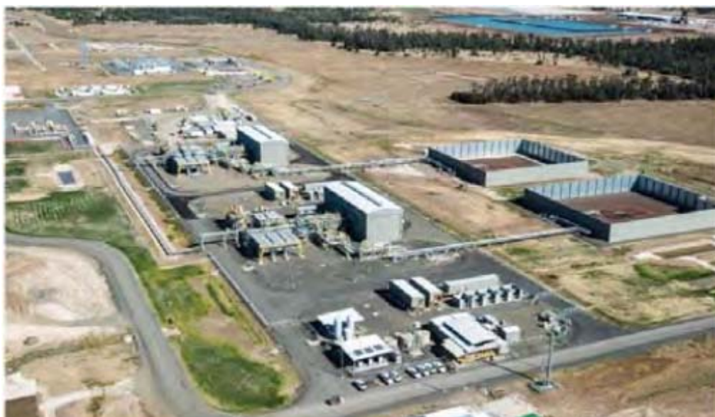
Condabri Central Gas Processing Facility
