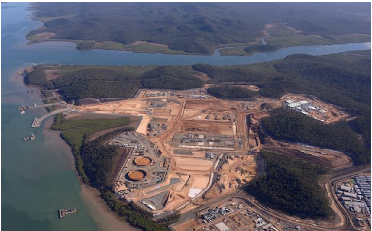
APLNG site on Curtis Island, October 2012
