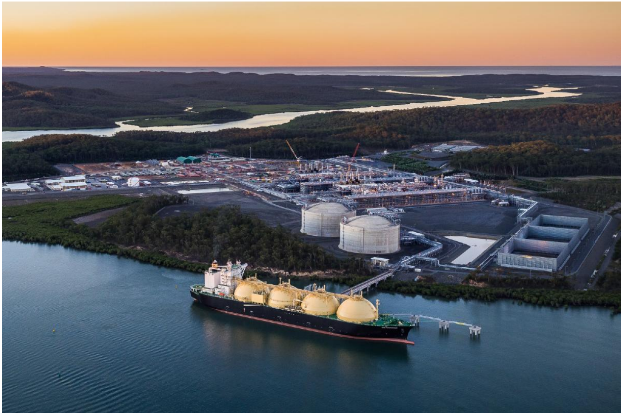
Australia Pacific LNG facility on Curtis Island
