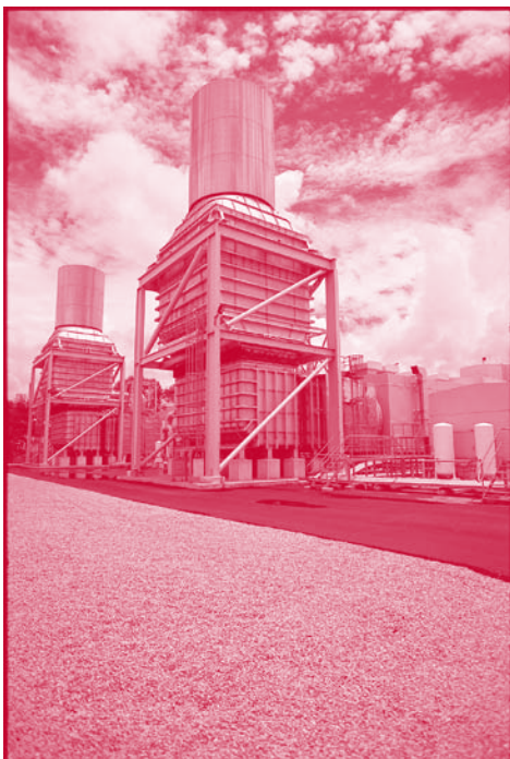
Electricity being generated at Queensland's Mount Stuart power station.
