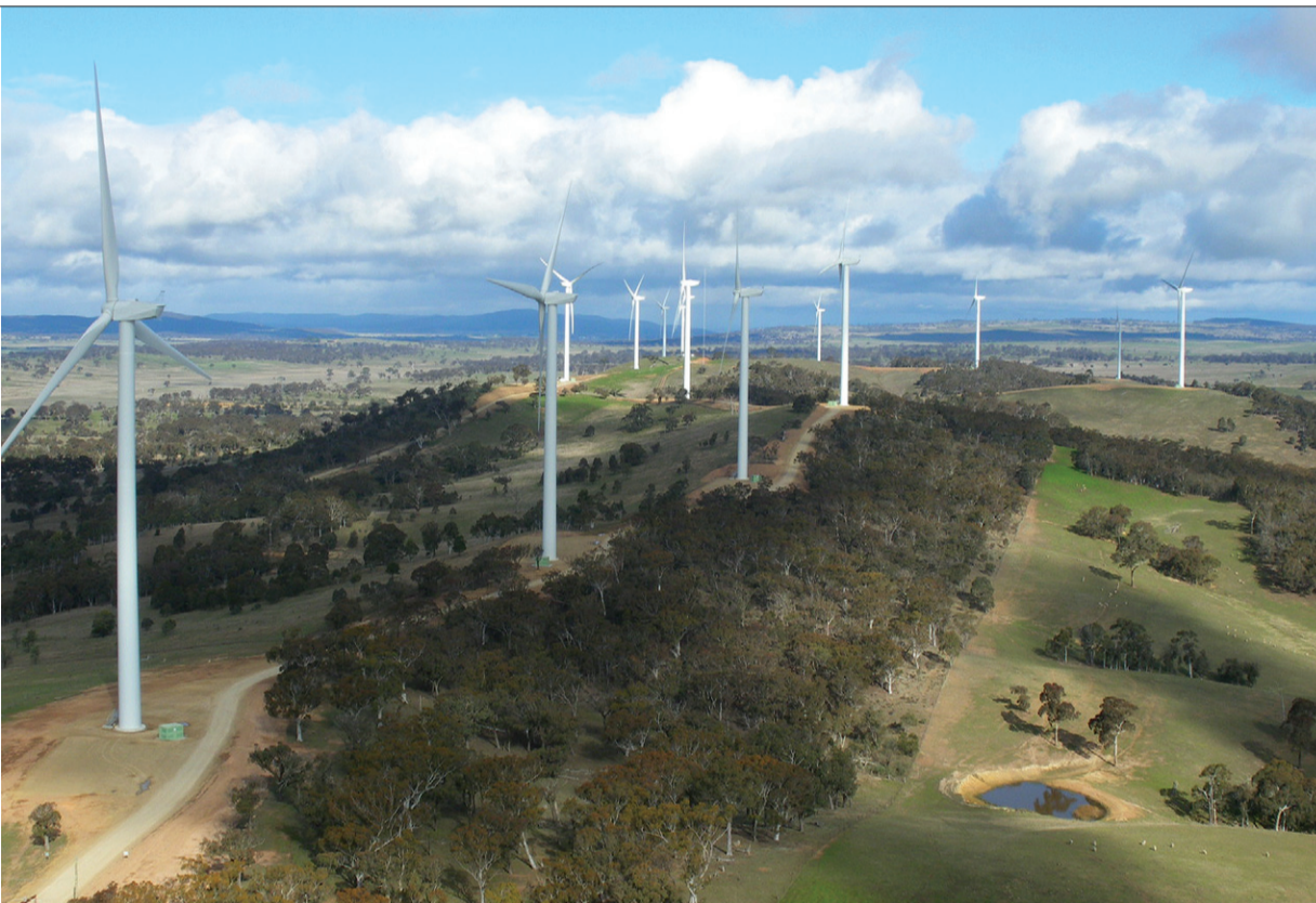
Energy harvested from the Cullerin Range wind turbines is fed into the NSW electricity grid. While wind power is an ancient form of energy, modern computer technology enables the wind turbines to adjust their angles according to the wind direction.
