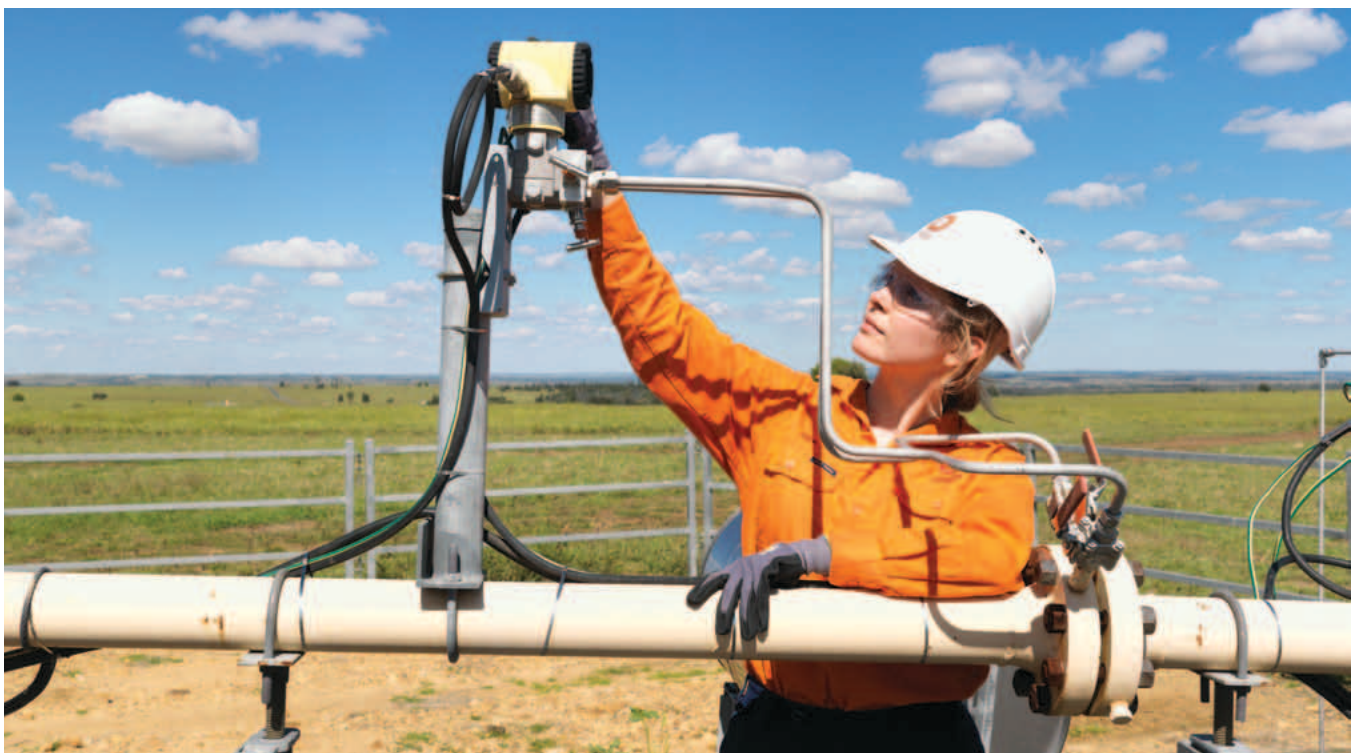
Checking a gas well at Spring Gully
