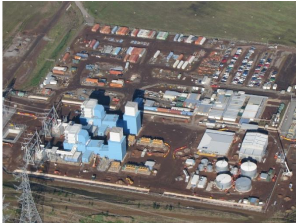
Aerial shot of Mortlake Power Station
