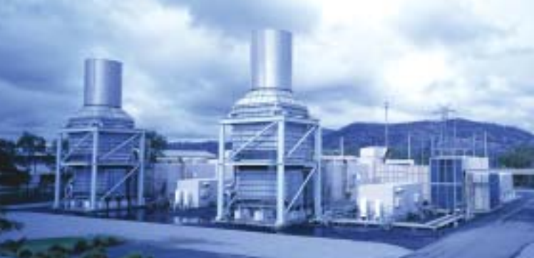
Mt Stuart Power Station, Queensland.
