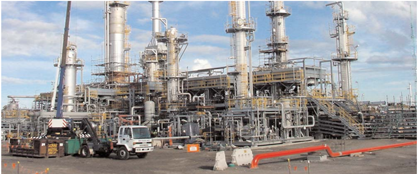
Figure 6: Example of construction of a production station (BassGas Project).
