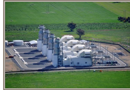
Uranquinty Power Station
