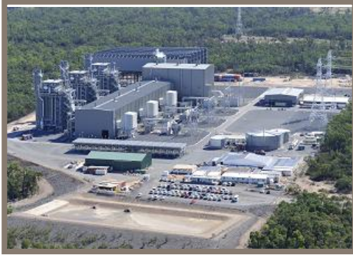
Darling Downs Power Station
