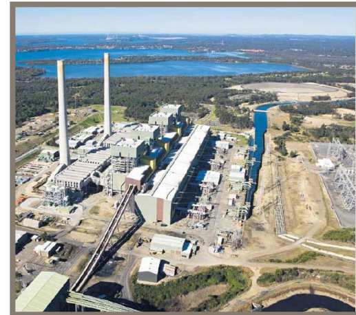
Eraring Power Station
