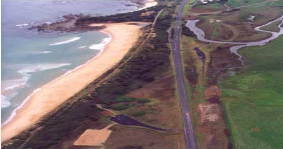
Shore crossing location at Kilcunda
