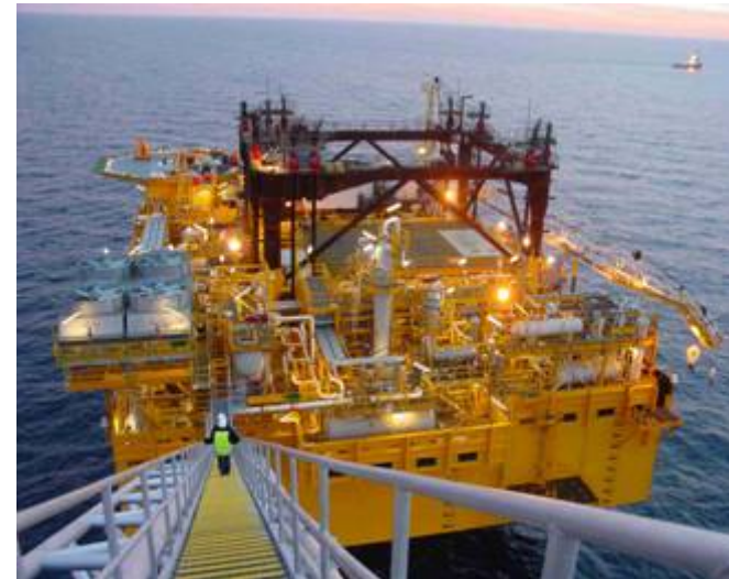
The Yolla A Platform, Bass Strait, during installation
