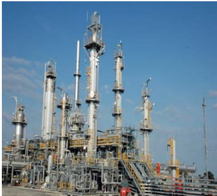
Onshore plant at Lang Lang, Victoria
