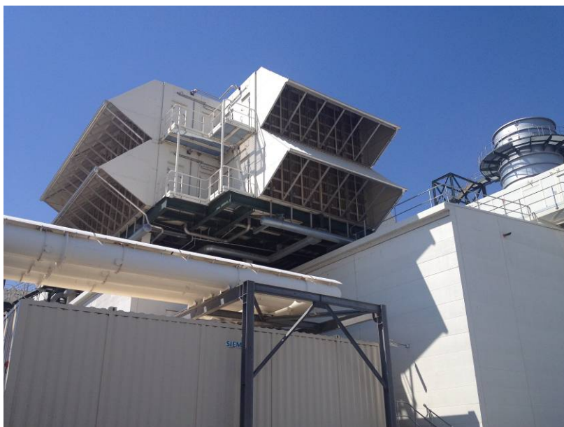
UPS Air Intakes
