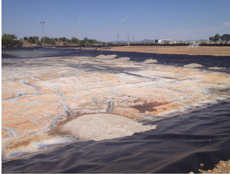
UPS Evaporation Ponds - Pond 1 emptied and solids removal occurring
