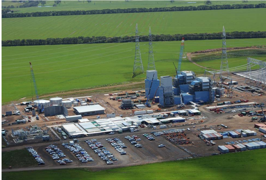
Aerial shot of Mortlake Power Station
